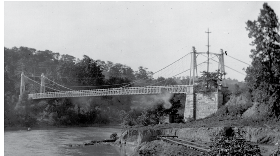
The suspension bridge over the Little Miami River at Beechmont Avenue, under construction about 1874.
