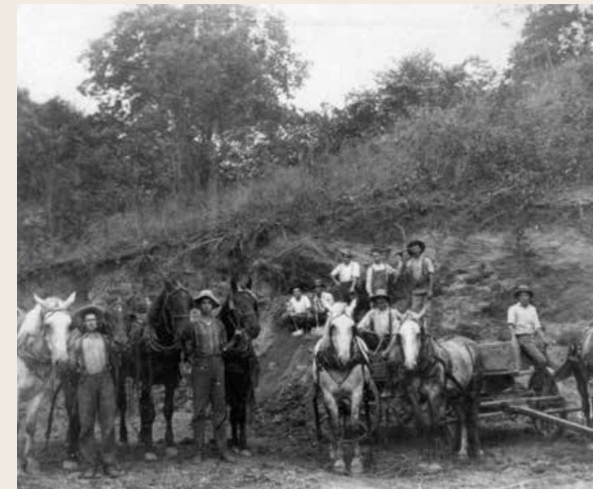
The newly purchased public roadway Clough Pike was in need of major repairs. Local farmers Clifford (second from left) and Charles (with the white horses) Wittmeyer were hired for road construction. The crew moved soil to fill in areas where the road was washed out. Photo from 1912.
