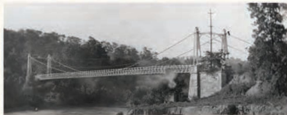
Beechmont Suspension Bridge, photo by Mary Shinn about 1910. Photos from the Anderson Township Historical Society Collections
