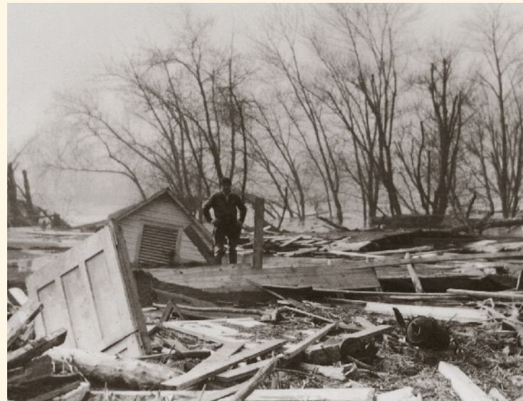
This photo illustrates the destruction of homes and businesses in California, Ohio, during the 1937 flood.
