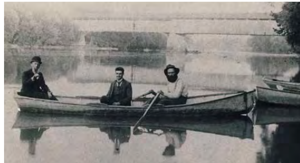
Men in canoe near the covered bridge over the Little Miami River.
