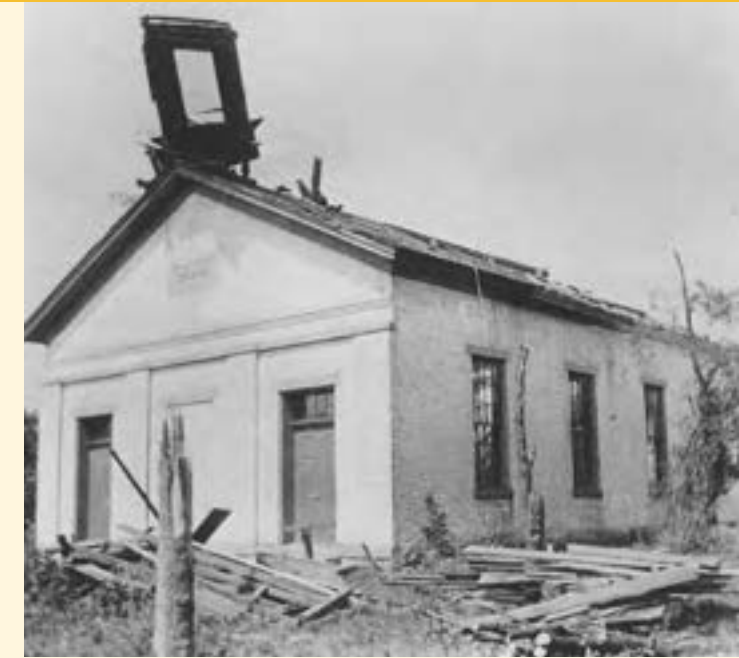
At Sutton and Corbly roads, the former Methodist Protestant Church lost its roof and steeple.
