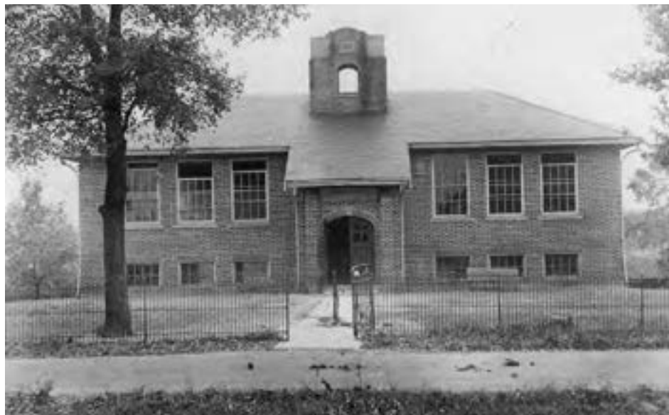
Cherry Grove School-southwest corner Eight Mile and Beechmont
