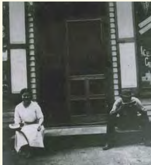
Outside Freda Vetter's drugstore, near southwest corner of Beechmont and Corbly, photo 1915.
