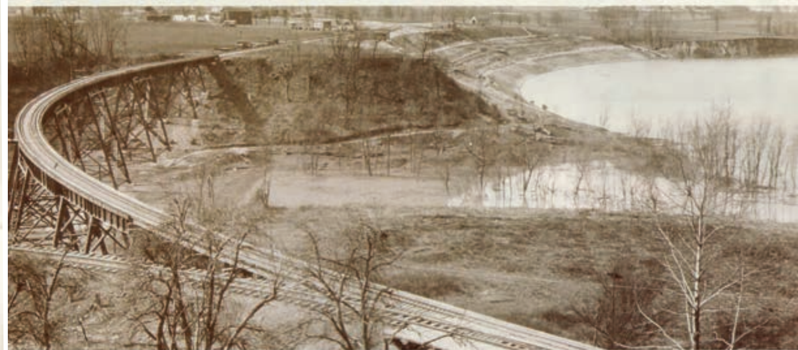
Rare view, looking east along the Ohio River, showing the tracks of the C. G. & P. over the Lick Run trestle to the Cincinnati Waterworks being built in California. The main line continued off to the left. Photo about 1900, when the C. G. & P. was still using narrow gauge track on main line and both narrow and standard gauge track on the new line to California.
