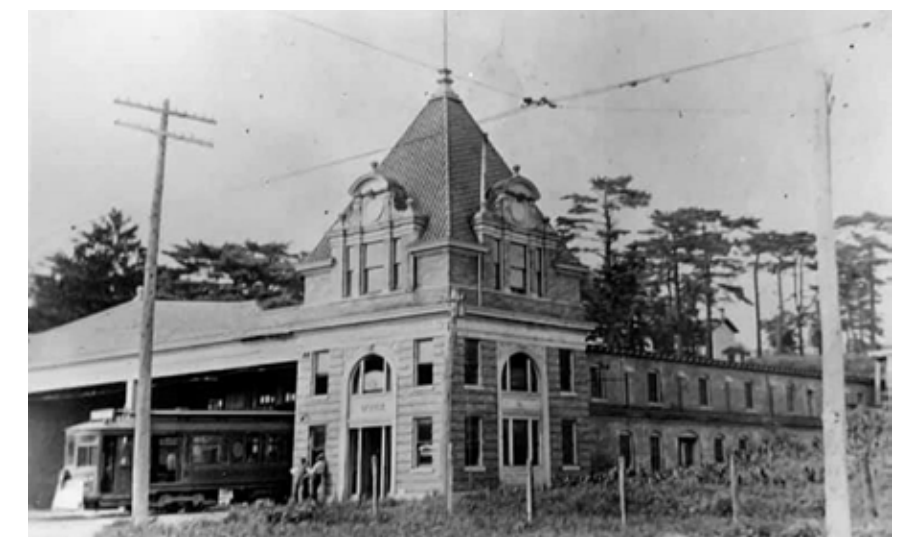
The IR&T power station and car barn located on the west side of Sutton Road across from Coney Island. From the Earl Clark collection.
