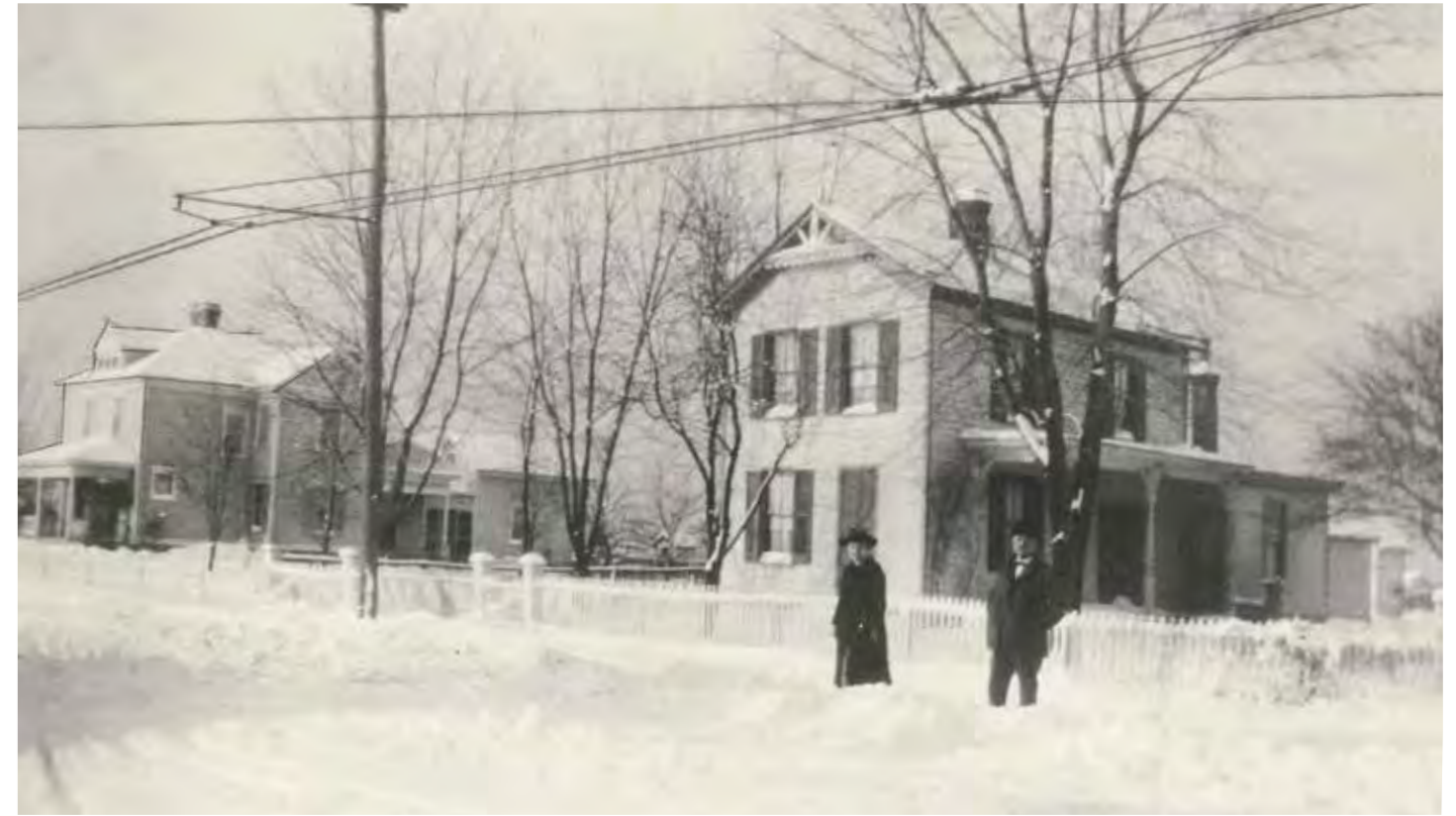
Waiting for the railway on snow-filled Beechmont Avenue in the winter of 1917-18. The house on left is the location today of Frisch's.
