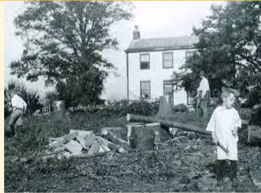
Shade trees around this house near Wayside were blown down. Photo by Ed Collord
