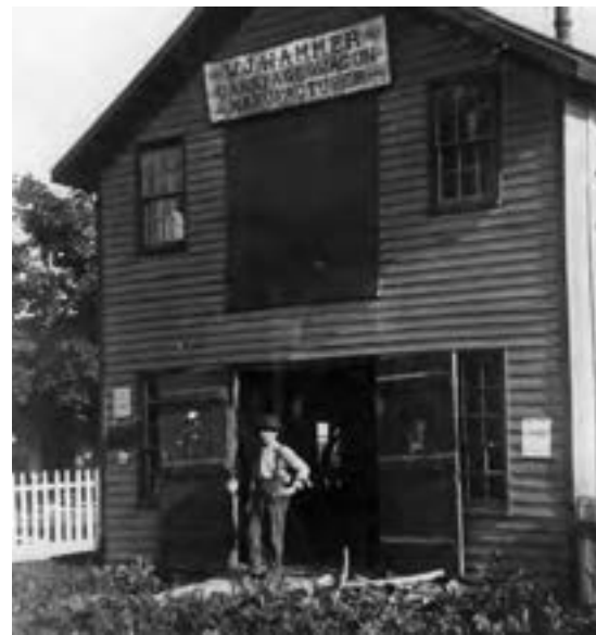
Hammer Carriage Shop-near Eight Mile and Beechmont in the Cherry Grove area
